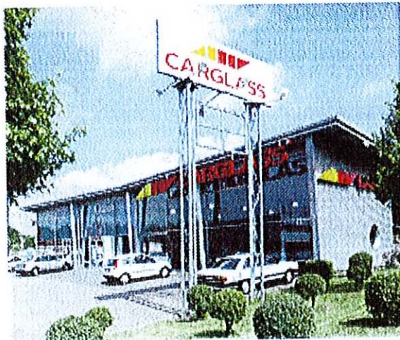
CARGLASS® Service-Center in Mönchengladbach-Wickrath: Adolf-Kempken-Weg 137
